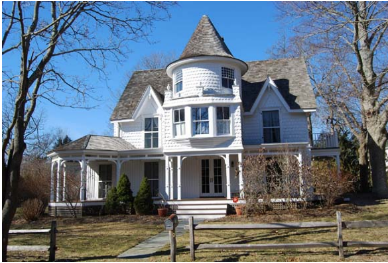
The Reed Cottage, circa 1870 at 25 Woodbridge Avenue
